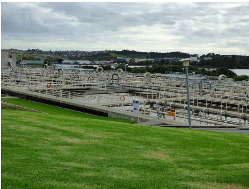
Rosedale Waste Water Treatment Plant
